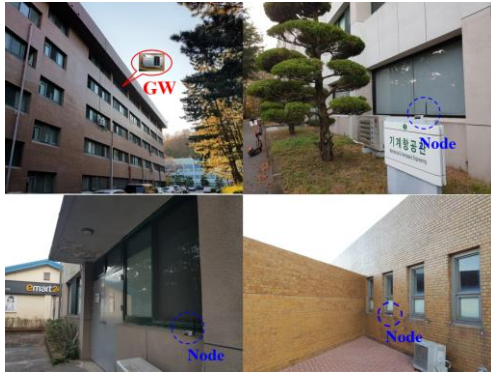
Fig. 5. Some spots of LoRa end devices
