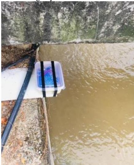
Fig. 16. Placement of sensor node underneath a bridge for river water level monitoring
