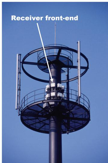
Figure 2. An example of a tower mounted RFE.
